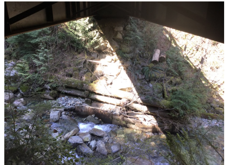
Left Bank Abutment when facing downstream
