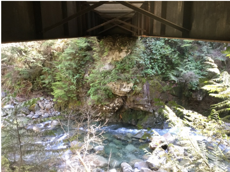
Right Bank Abutment when facing downstream
